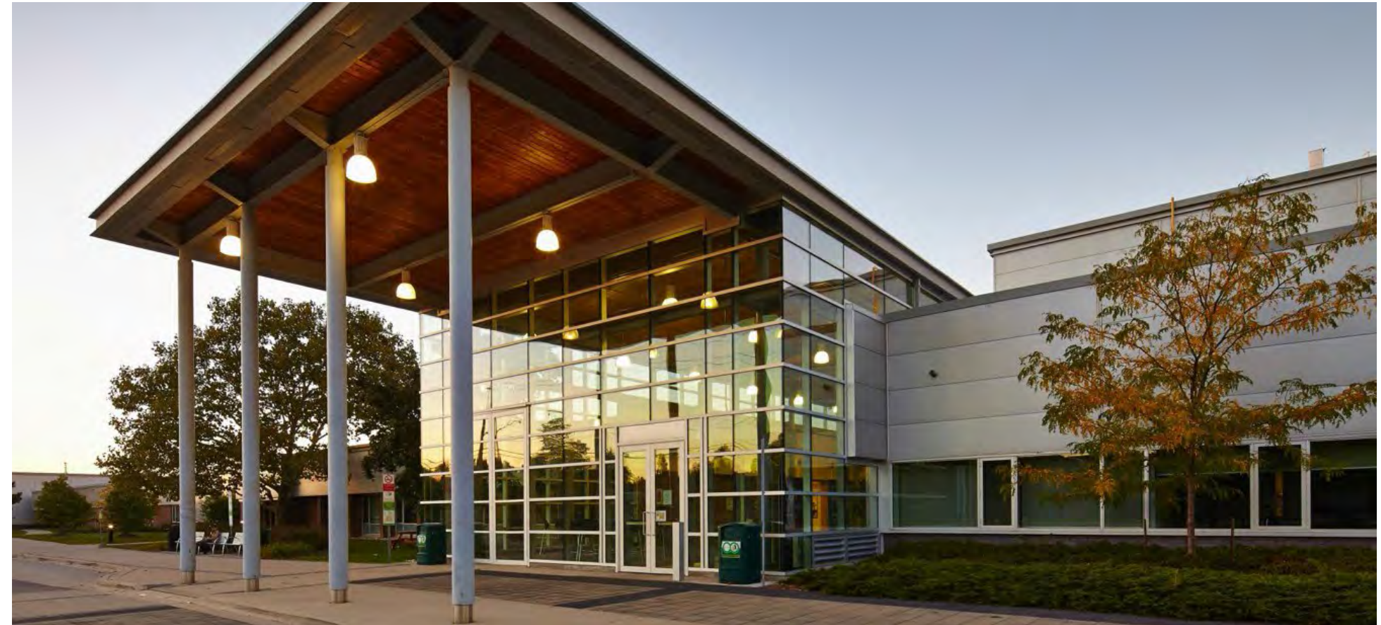
The existing entrance to campus provides opportunities for enhancement.
