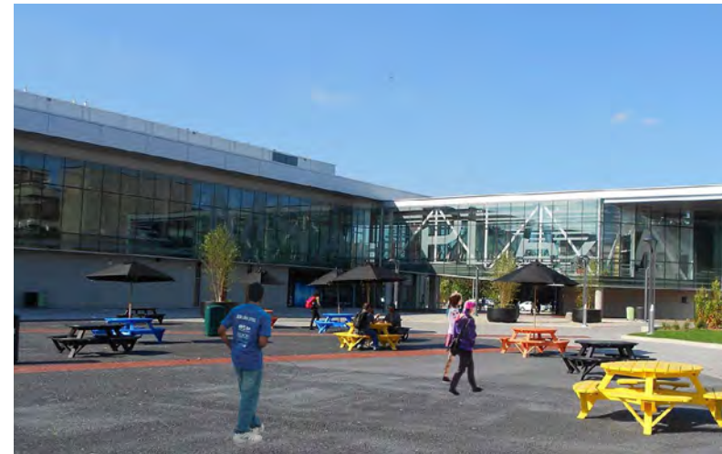
The plaza lacks a purpose in winter. A skating rink, which was originally contemplated during the design of the plaza but cut due to budget constraints, would create activity for this centrally located public plaza during cold weather months.
