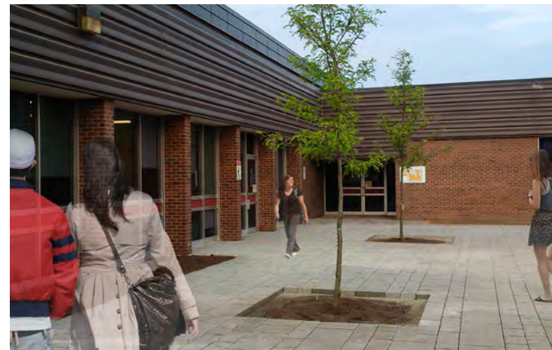
The current state of the Courtyard.
