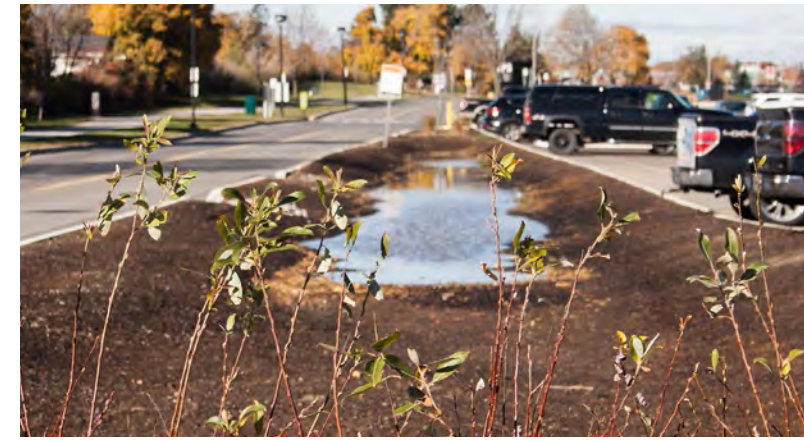
Current - bioswale located off of Governors Boulevard, Fennell Campus.
